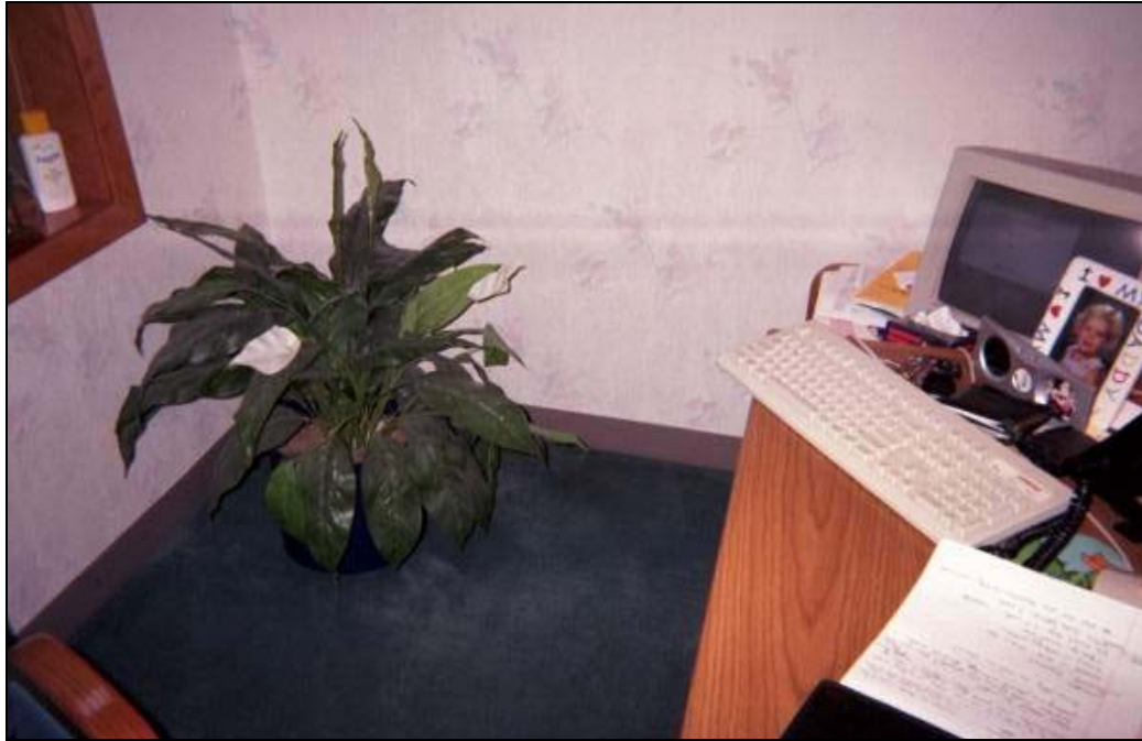
Photograph 3 Office Area where Carpet got Wet
